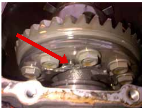
Figure 6 Broken bolts and flange
